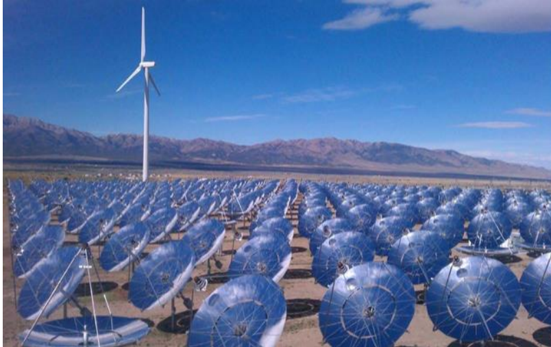
Figure 4. A portion of the Infinia 1.5 MW dish Stirling installation at Tootle Army Depot
