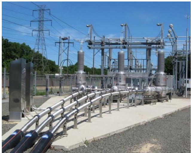
Figure 20. AMSC 3-phase AC HTS distribution line emerging from the ground to transition to conventional power lines (Courtesy of AMSC)
