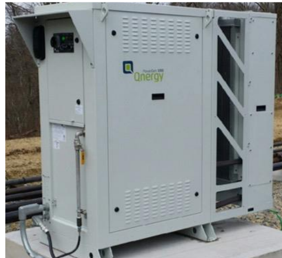
Figure 19. Qnergy PowerGen field installation
