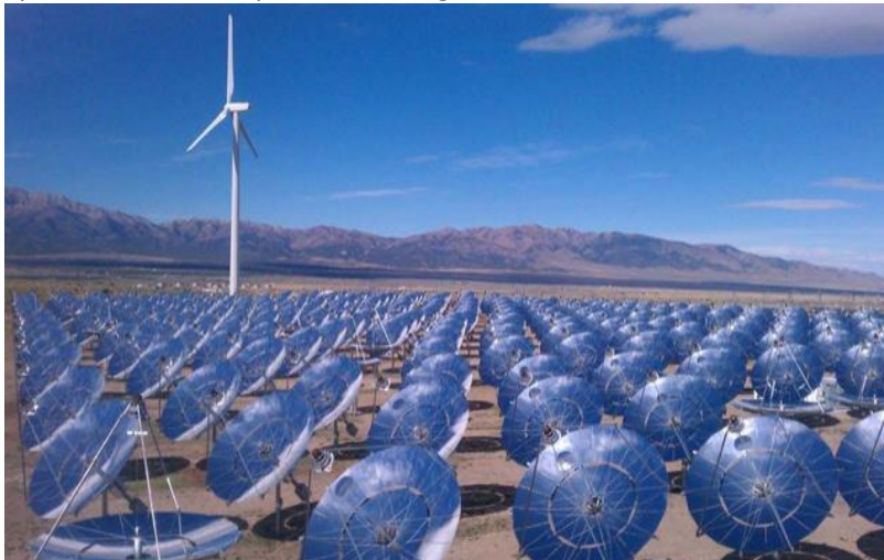
Figure 4. A portion of the Infinia 1.5 MW dish Stirling installation at Tooele Army Depot
